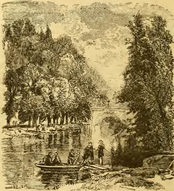
BRIDGE AT VALLEY GREEN.
